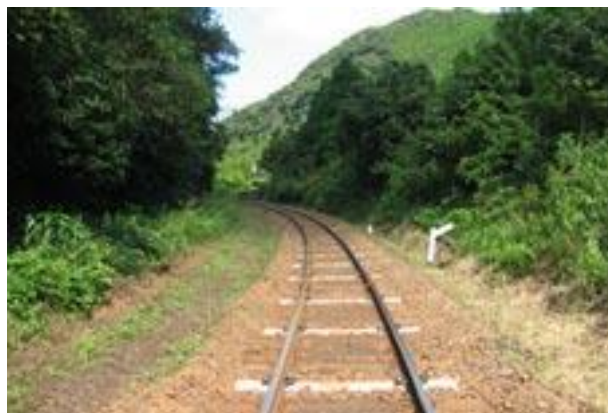
Figure 24: Example of TPC sleeper installation 44
